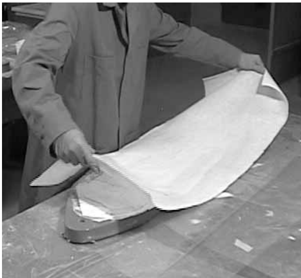
9. Place perforated film and breather fabric over the release fabric. Perforated film restricts the amount of epoxy that can be drawn away from the lay-up into the breather fabric.
