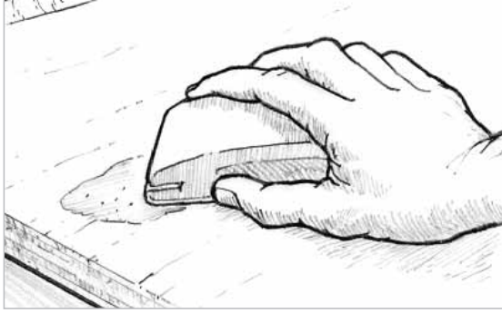
Figure 5-16 Sand the fairing material to blend with the surrounding contour.
